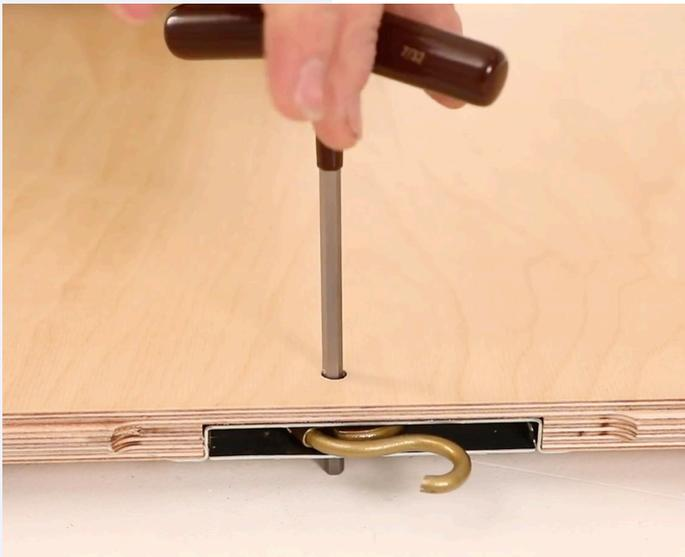
Lay the first panel of the second row (panel E) and latch it to the first panel of the first row (panel A), using the latching tool supplied. Ensure that each latch is fully retracted by turning the key first in an anti-clockwise direction until you hear a click, then turn it fully in a clockwise direction to engage it in the receiver. If panels are aligned correctly, the latches engage easily.
