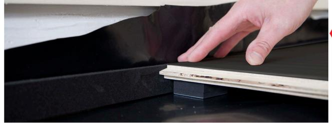
Use spacer blocks to fix the panels 10mm from the wall, or fit the optional plastazote strip.
