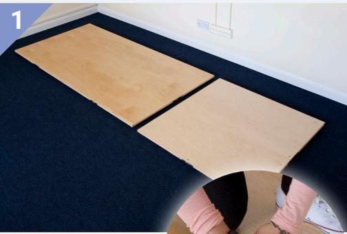
Place your 1m x 1m and 2m x 1m Harlequin Liberty® sprung floor panels onto your sub-floor. Push the smaller panel against the larger panel and join them together using the locking tool. You will need to turn the locking tool a full 360 degree revolution and will hear a noticeable 'click' once the latch and lock mechanism has joined together.
