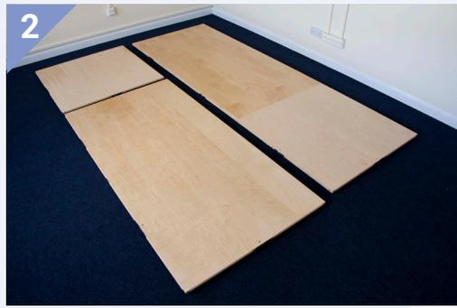
Place your other 1m x 1m and 2m x 1m Harlequin Liberty® sprung floor panels onto your sub-floor, so that they are in a brickwork layout. Push the panels against the other panels and join them together using the locking tool.
