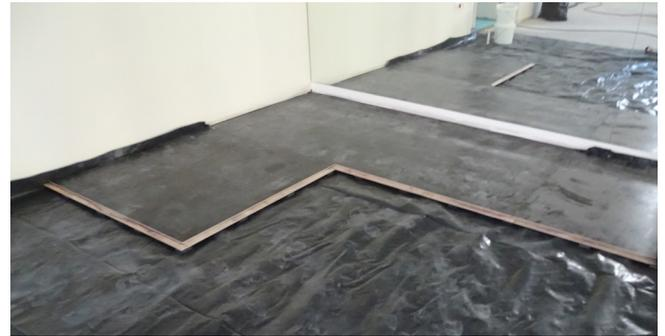
If your room is exactly the same as a row of panels, or the off-cut piece is less than 300mm, then the second row should start using a panel sawn in half.
