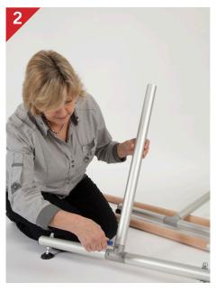
2. Tighten the hex screws with the Allen/hex key provided.
