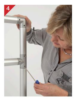
**4.** Tighten the hex screws with the Allen/hex key provided.
