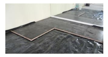
If your room is exactly the same as a row of panels, or the off-cut piece is less than 300mm, then the second row should start using a panel sawn in half.
