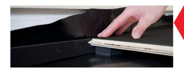
Use spacer blocks to fix the panels 10mm from the wall, or fit the optional plastazote strip.
