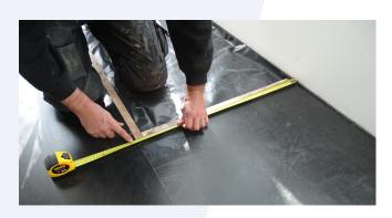
Cut a panel to this exact size, removing the pads if required and sandpaper any rough edges. Retain the remaining piece of the panel for use as the start of the second row.
