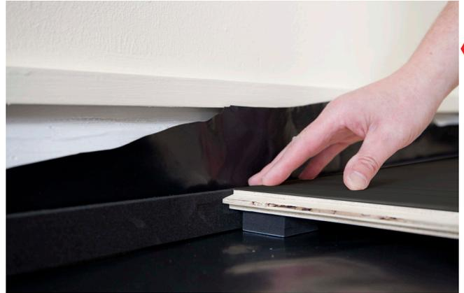
Use spacer blocks to fix the panels 10mm from the wall, or fit the optional plastazote strip.
